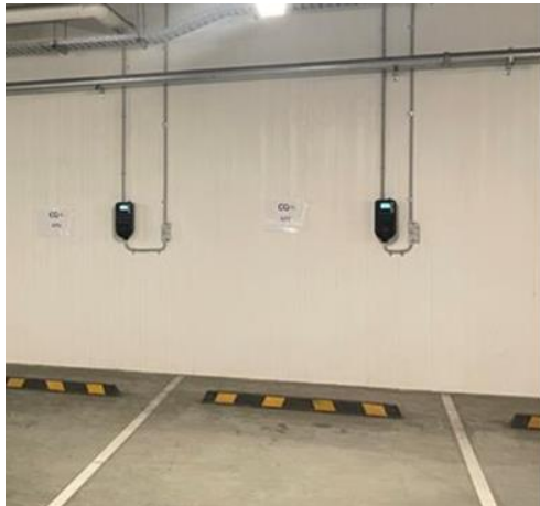
Car spaces with EV chargers installed
