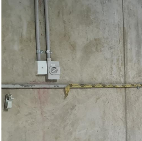
'EV Ready' car space with power and communications cabling
